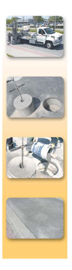
1. The coring truck sets up and cores up to an 18" diameter hole up to 22" deep in the sidewalk or roadway in minutes.
